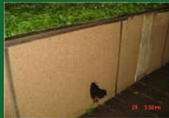
Air leaks - chamber side
